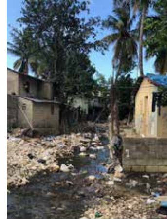
Damage from Hurricane Matthew, Dominican Republic
