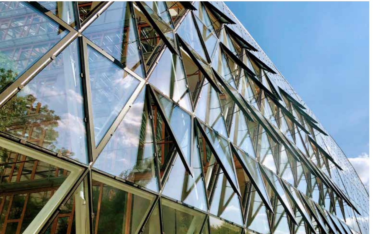
EIB/EKI building. Author: Paolo Gambino, EIB employee
